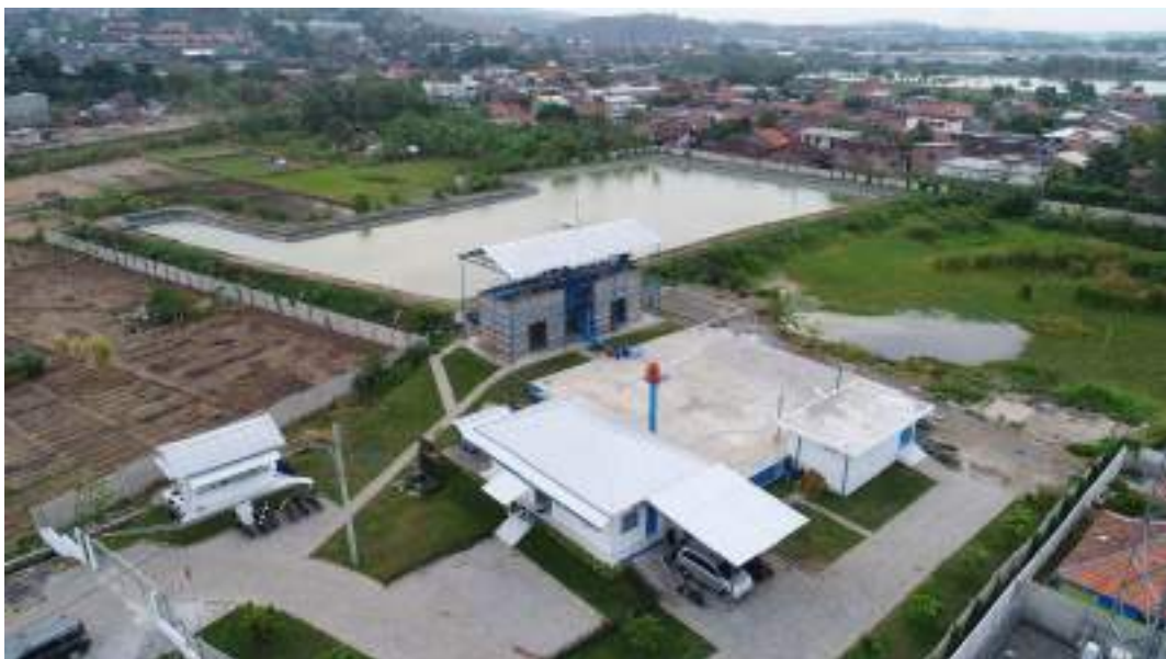
Gambar 8 Water Treatment Plant
